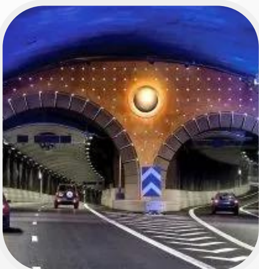
Marine Drive - Orange Gate tunnel
