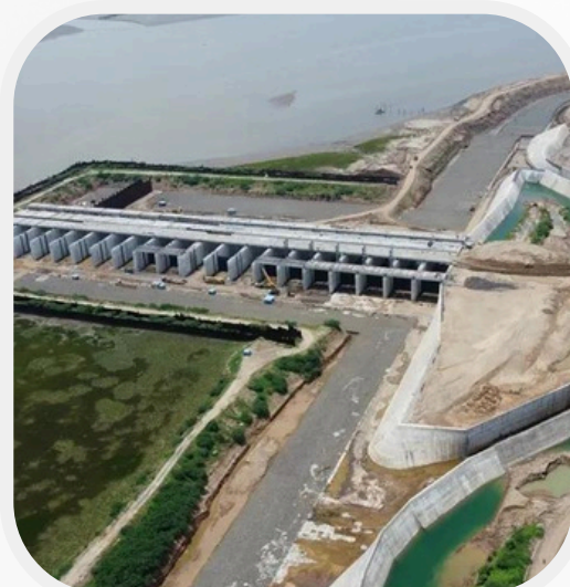
Bhadbhut Barrage Project
